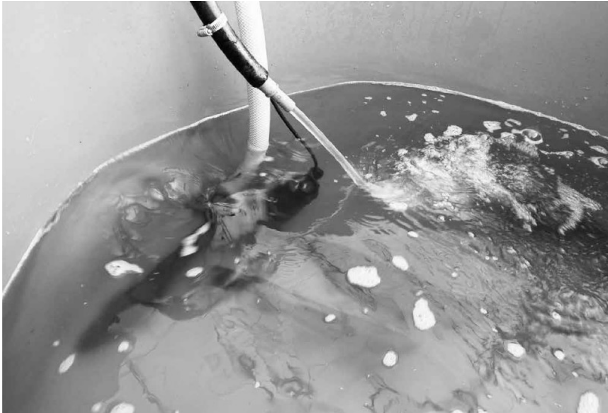
Purge tank with submersible pump for aeration and circulation.
