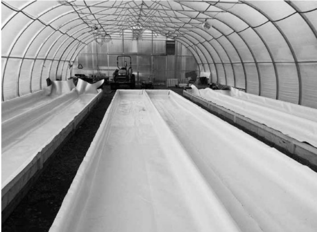
Nearly completed trough liner installation.
