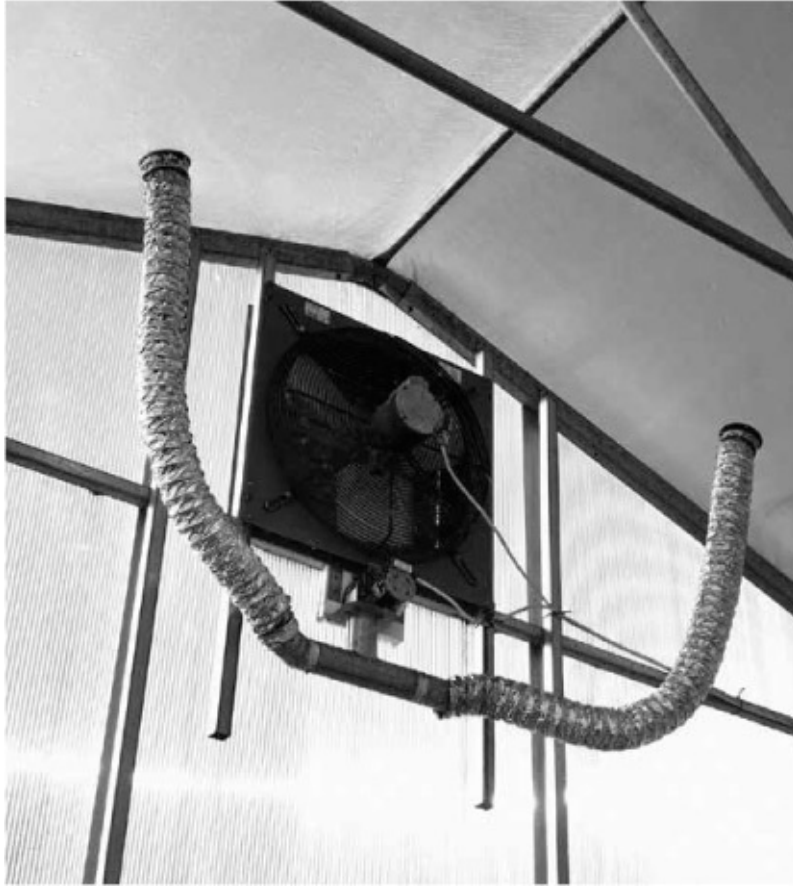
Peak vent and double-layer poly inflation blower.
