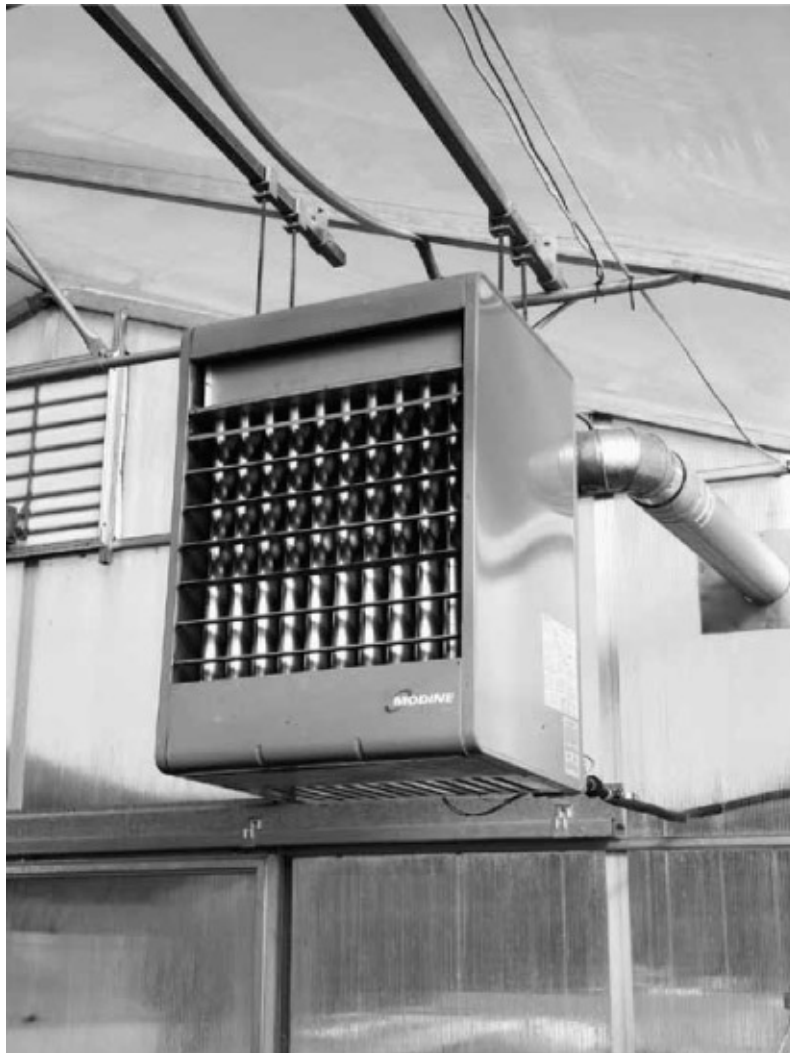
Vented propane greenhouse heater.
