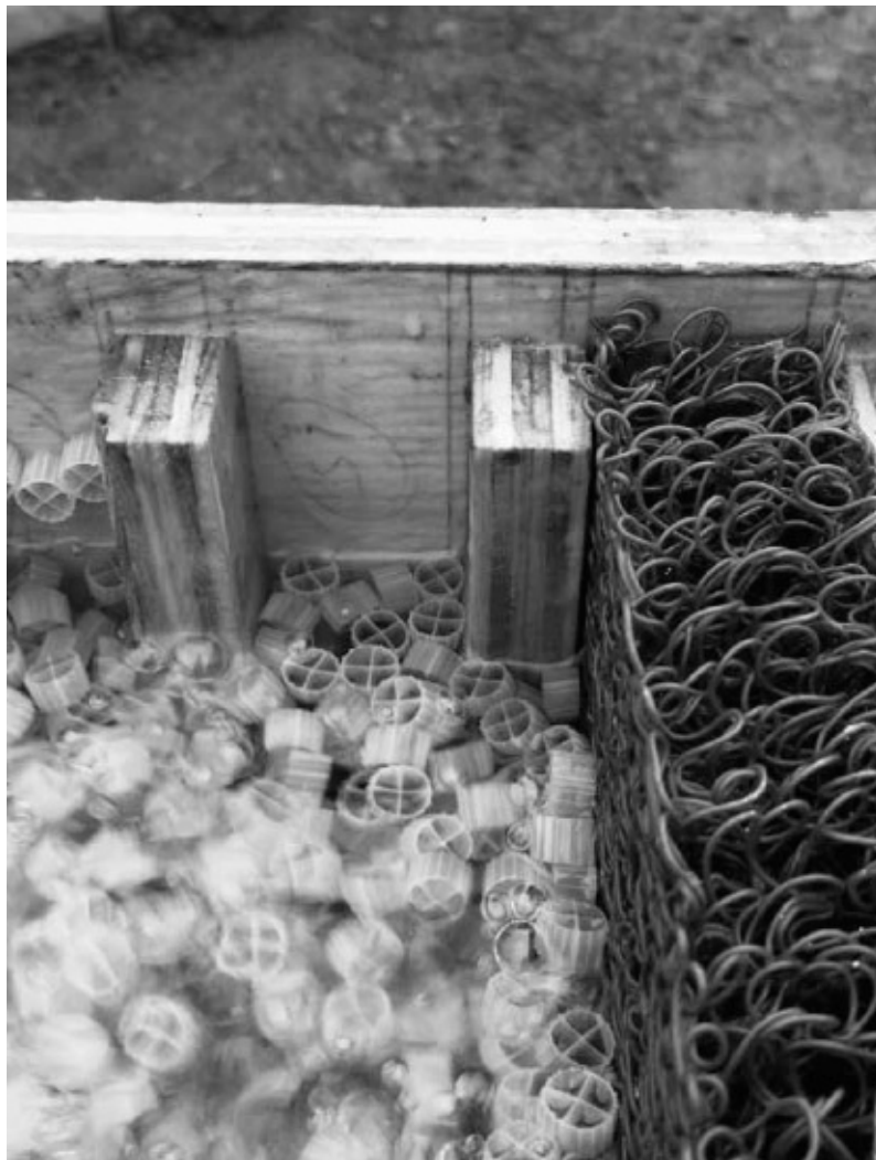
Filter screen (right) and MBBR media (left) in the CFB.
