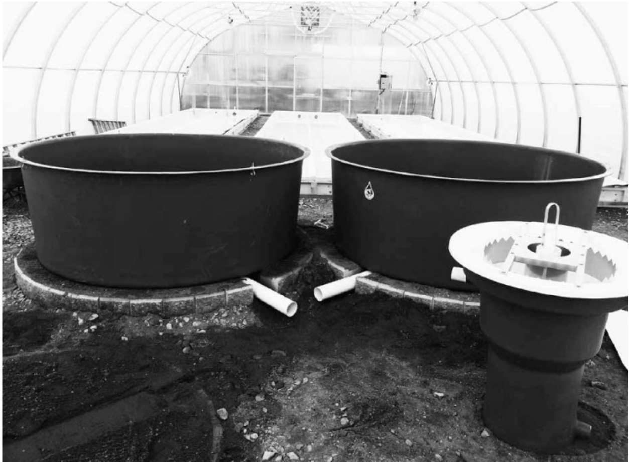
Tanks 2 & 3 on bases with roughed-in plumbing and RFS.
