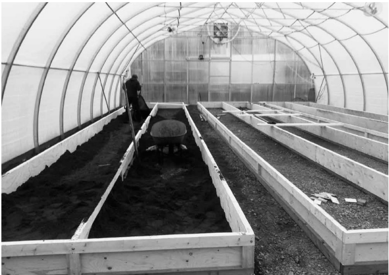
Laying the sand base in newly constructed troughs to protect the LDPE.
