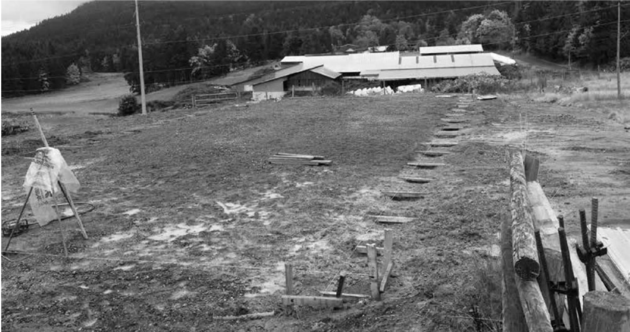
Foundation installation with string lines and batter boards, ready for concrete piers.
