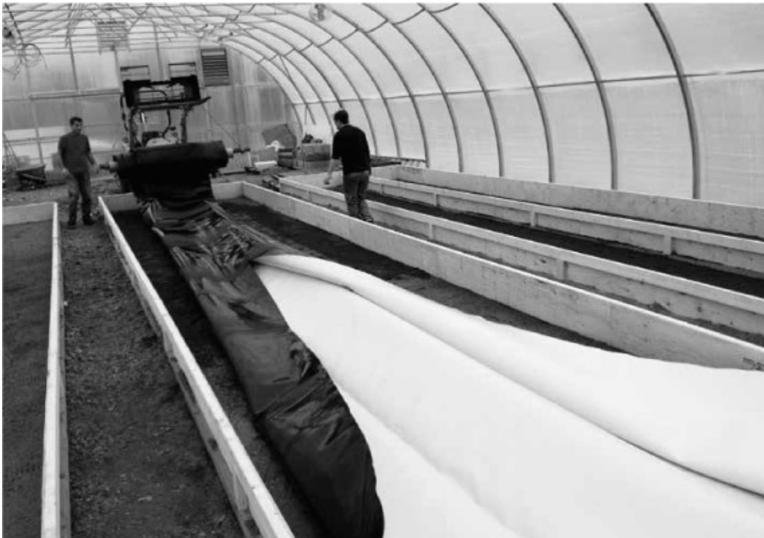
Rolling out the LDPE for liner installation.
